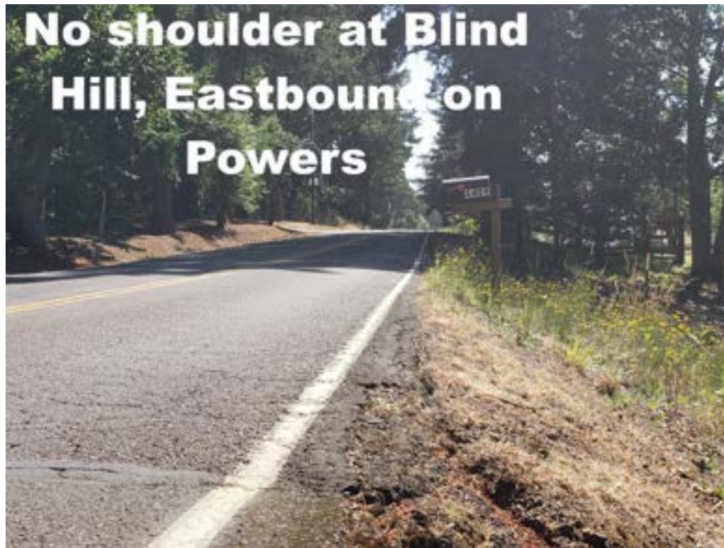
Figure 4. No shoulder, pedestrians, a blind hill, and high-density event traffic is a recipe for disaster.
